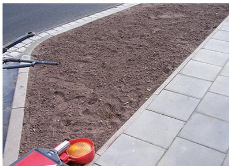
Fig. 8. Filling with Hydralit structural soil (Szczecin city, source: [www.tegra-polska.pl](http://www.tegra-polska.pl))
