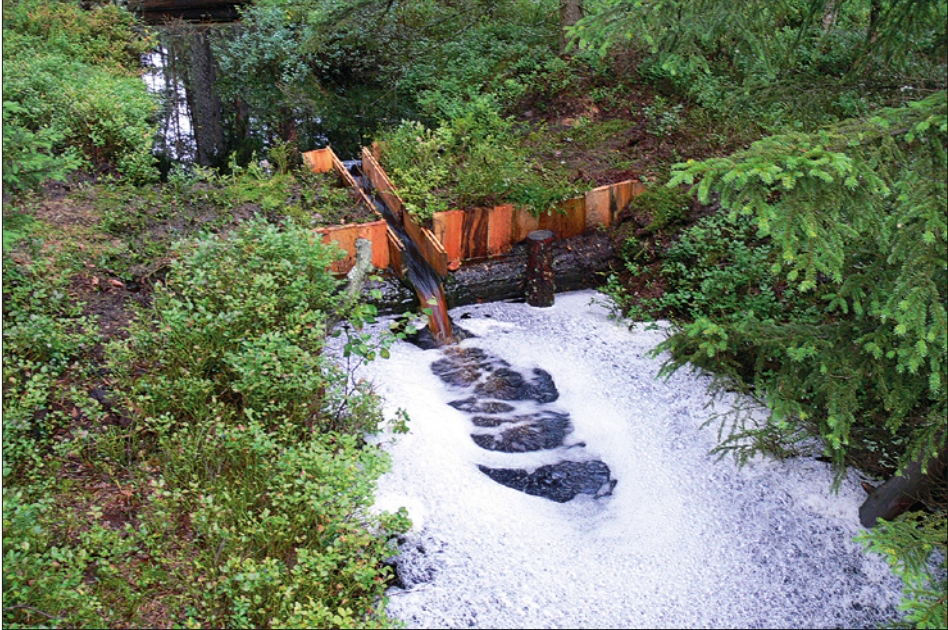
Figure 6. Gate in the “Staniszewskie Błoto” nature reserve built in 2007 under the project of peat bog active protection (photo by Jacek Herbich)
